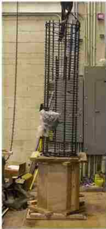
a). Column reinforcement
