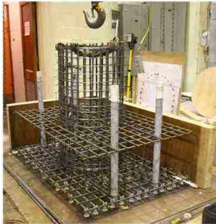
b). Shaft-Footing reinforcement
